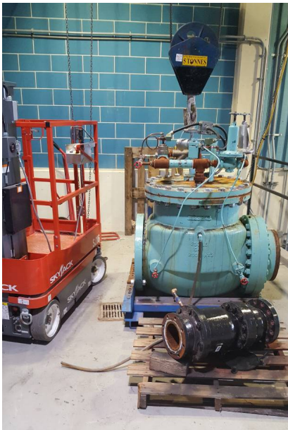
Figure 7a: Discharge piping showing location where high lift control valve was removed.
