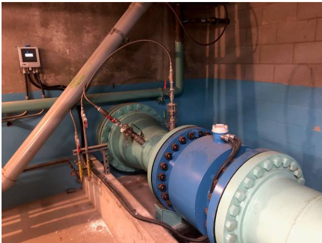
Figures 5a and 5b: New flow meters installed on the east and west treated water lines. The flow meter readouts are mounted on the wall.
