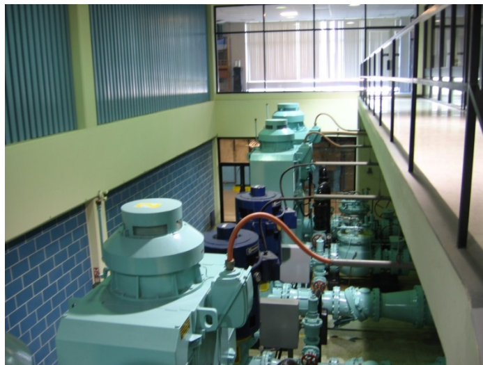
Figure 1: High Lift Pumping Station at WTP
