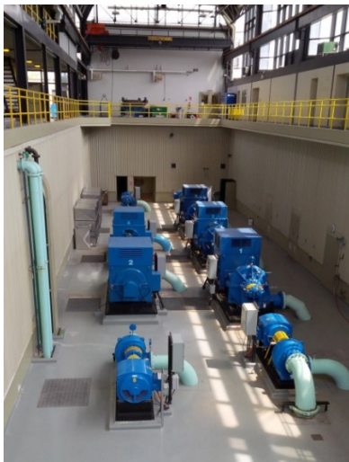
Figure 1: High Lift Pumping Station at WTP
