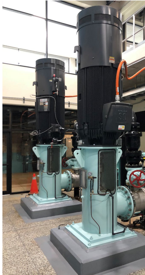
Figures 4a & 4b: New 500hp High Lift Pumps #1, #2, #3 & #4 in the High Lift Pumping Station.
