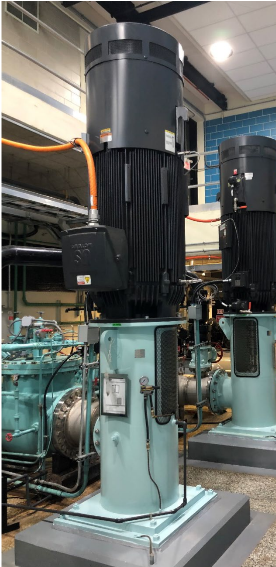
Figures 4a & 4b: New 500hp High Lift Pumps #1, #2, #3 & #4 in the High Lift Pumping Station.
