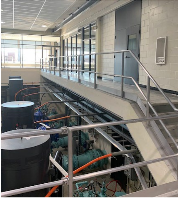
Figures 8a & 8b: New safety railings in the high lift pump gallery and stairwell.
