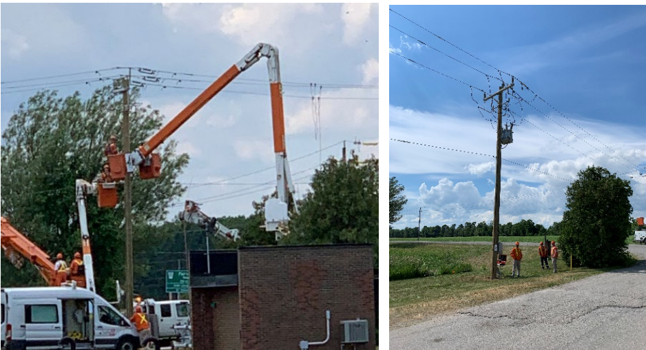
Figures 7a & 7b: WTP incoming power feed pole replacement.
