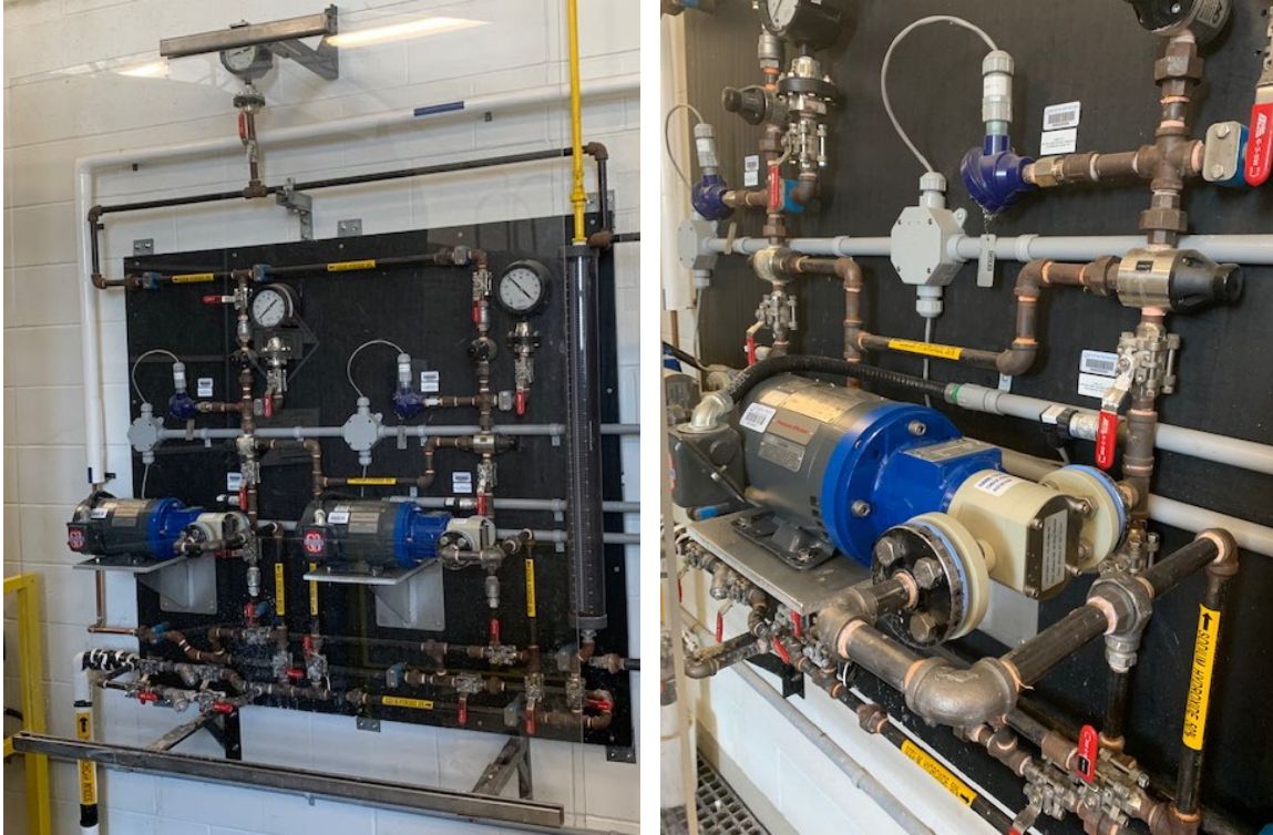
Figures 6a & 6b: New sodium hydroxide chemical dosing pumps.
