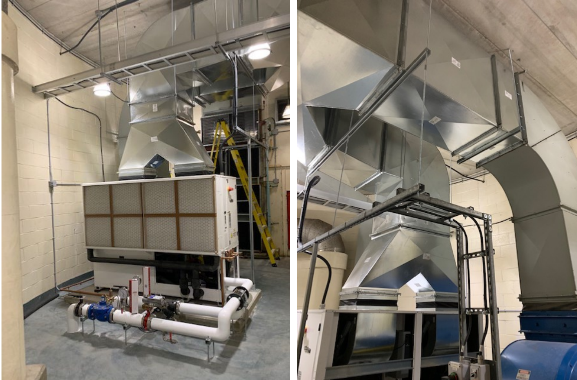
Figures 5a & 5b: New heat pump unit in the Mechanical Room at the Low Lift Pump Station.
