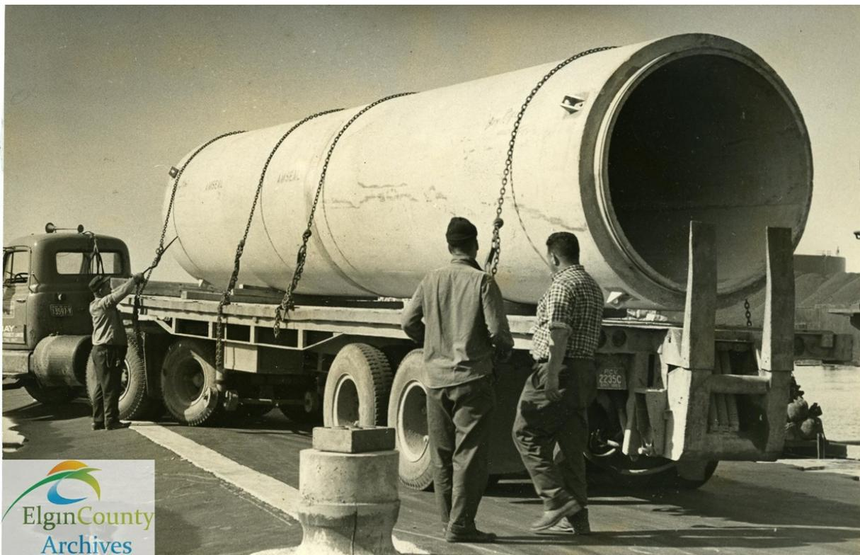
(1966) The first pipe arrives at the water treatment plant for the 60-inch diameter pipeline between the intake crib and the low lift pump station. ~ St. Thomas Times Journal
