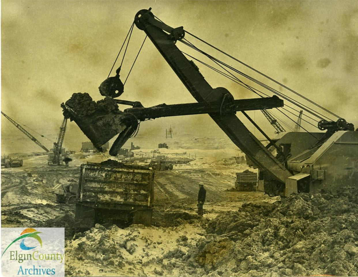
(1967) "In the midst of high winds and driving snow men and machines continued to move the earth at the site of the Lake Erie water supply system east of Port Stanley. Installation of steel pilings for the base of the low lift pumping station has been carried out and cliffs surrounding the site are still being graded." ~ St. Thomas Times Journal
