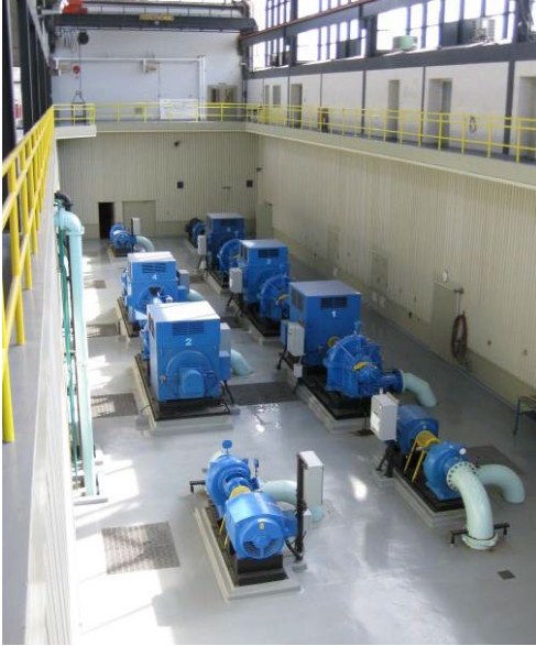
Figure 2: High Lift Pumps at the Lake Huron WTP
