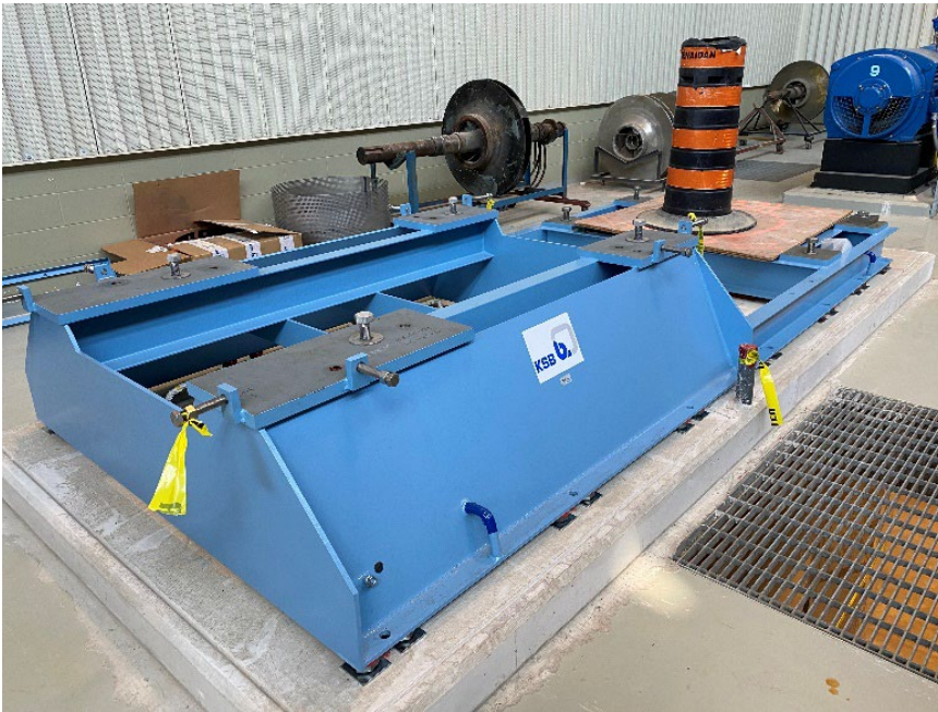
Figure 7: New HLP #6 pad and pump base plate (August 2021)
