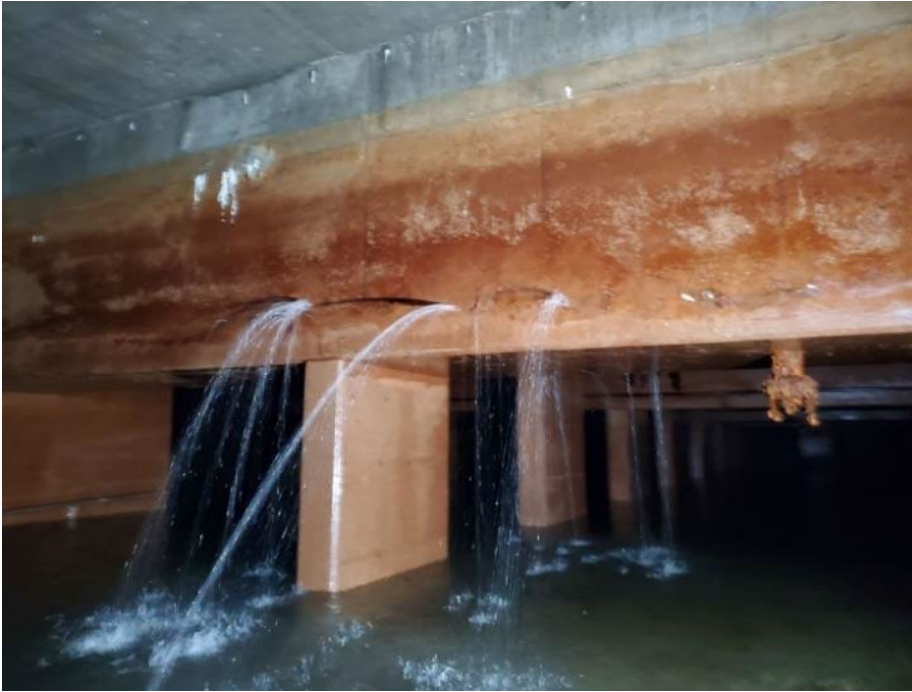
Figure 10: GMBP inspection photo showing leakage (before repair); Location is Filter #8 - east face north of baffle wall
