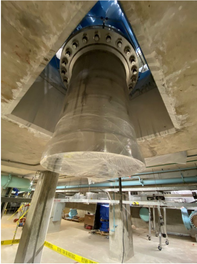
Figure 9: The spool piece for HLP #5 is installed in the pipe gallery below (October 2021)
