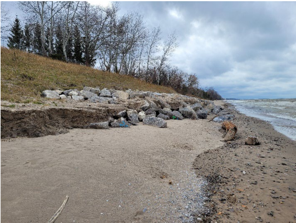
Figure 15: Post-construction photo from December 2021. The beach chamber is fully protected by armour stone.
