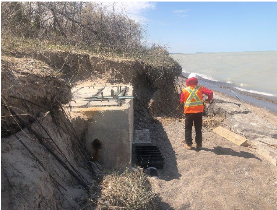
Figure 13: Pre-construction photo from May 2020 showing further erosion impacts and exposure of the beach chamber.
