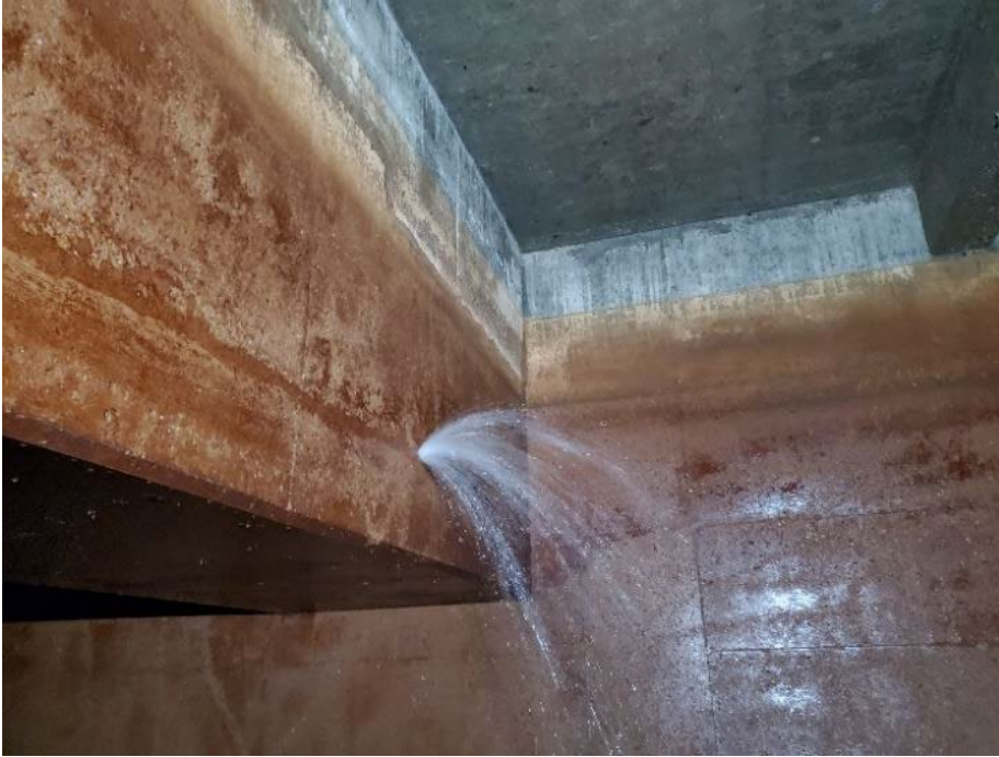
Figure 11: GMBP inspection photo showing leakage (before repair); Location is Filter #10 conduit - west face north of baffle wall
