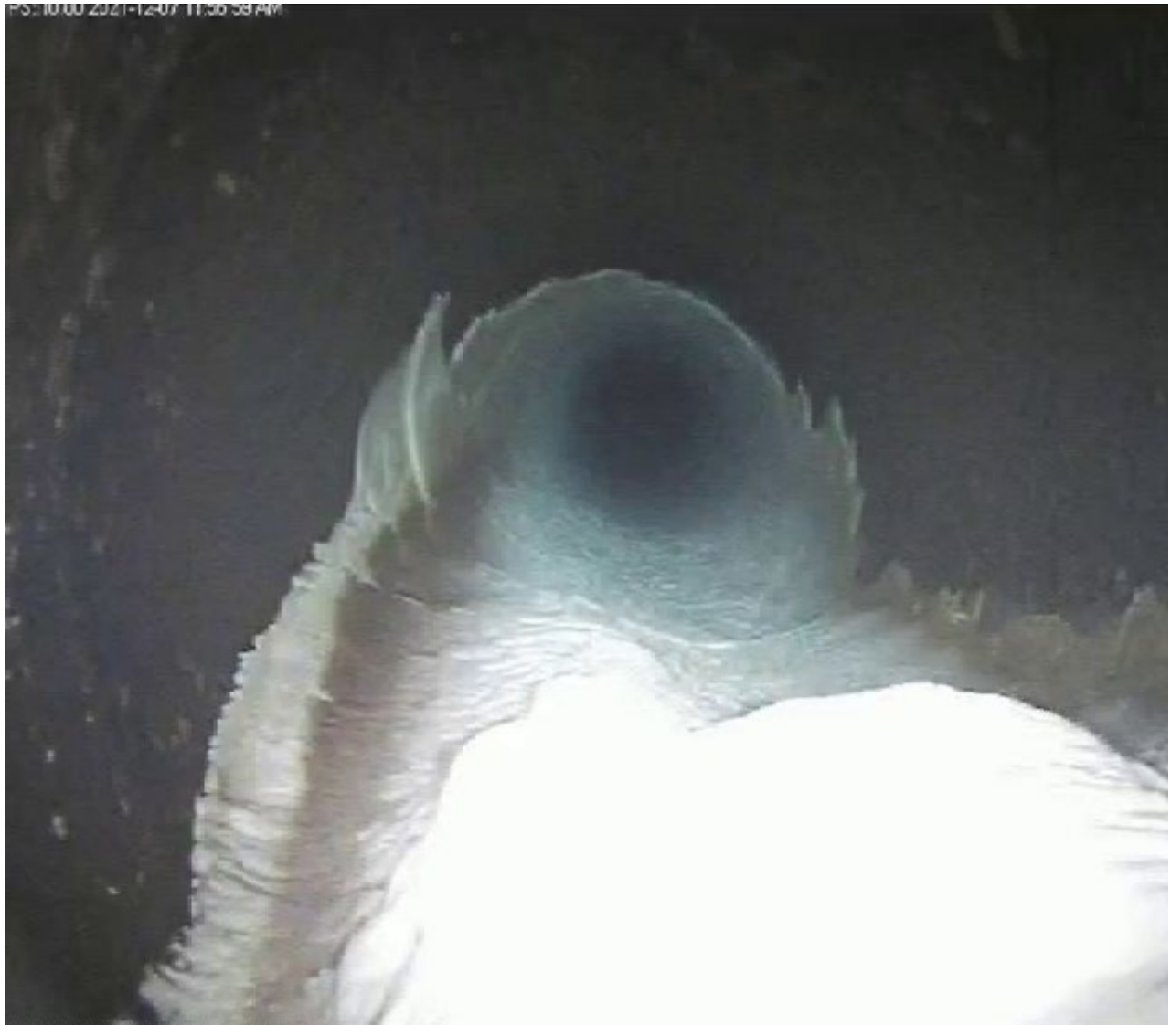
December 2021: Looking downstream from the sodium hydroxide injection showing the precipitate accumulation in west discharge header
