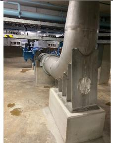
Photo 7: High lift pump pipe gallery showing new high lift pump 5 discharge piping, control valve and isolation valve
