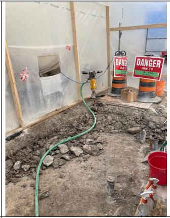
Photo 2: Inside dust containment area showing progress of removal of pump 3 base
