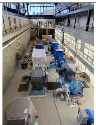
Photo 1: High lift pump gallery showing from back to front, existing pumps 1, 2, 3 (removed with dust containment area) and pumps 4 (existing) 5 (small new) and 6 (large new)
