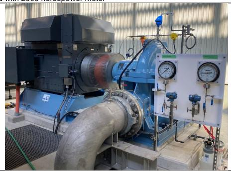
Photo 4: New high lift pump 6 (large) installed in the spare slot rated at 1300 litres per second at 150 metres total dynamic head with 3500 horsepower motor
