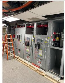
Photo 8: High lift pump electrical room showing installation of motor control centre that supply power to the high lift pump motors 1, 2 and 3
