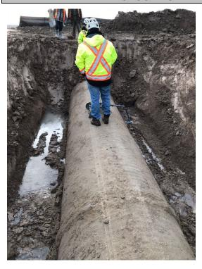
External Electromagnetic Verification of the Pipe
