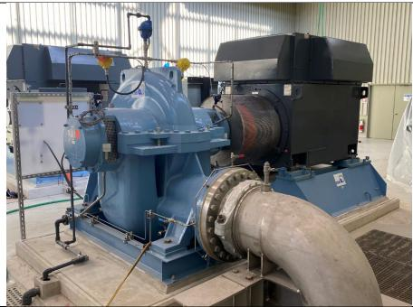
Photo 3: New high lift pump 5 (small) rated at 900 litres per second at 125 metres total dynamic head with 2000 horsepower motor
