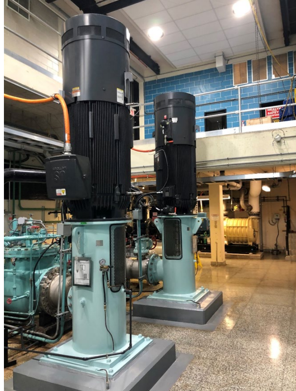
Figures 1a & 1b: New 500hp High Lift Pumps #1, #2, #3 & #4 in the high lift pumping station
