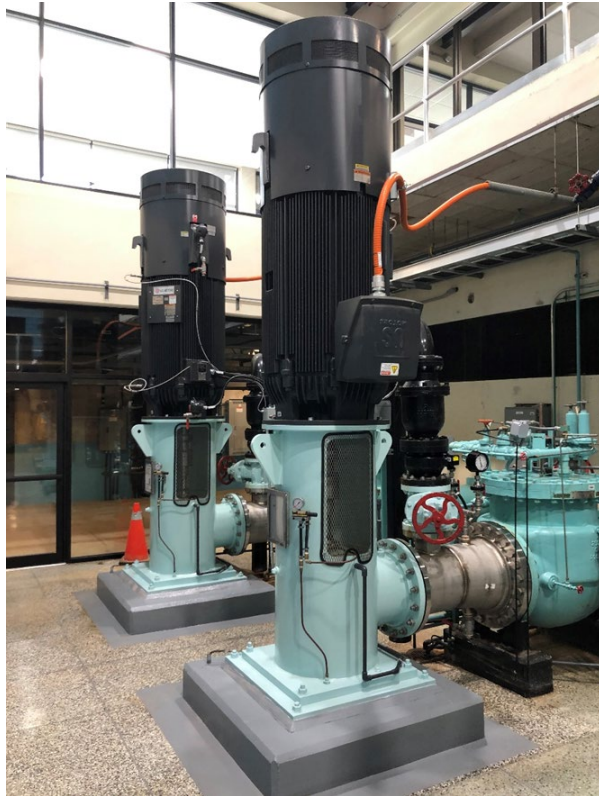
Figures 1a & 1b: New 500hp High Lift Pumps #1, #2, #3 & #4 in the high lift pumping station
