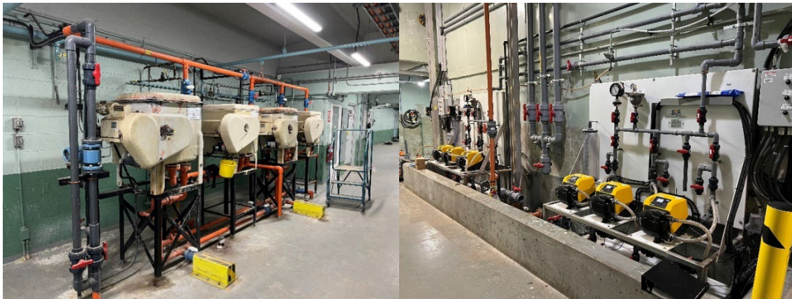
Figure 4a: The four (4) original rotodip wheel-type chemical feeders which are scheduled for decommissioning
