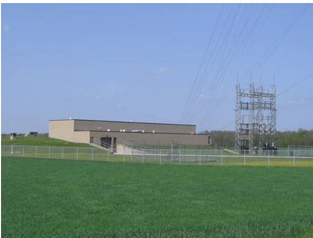
Figure 1: McGillivray Booster Pumping Station
