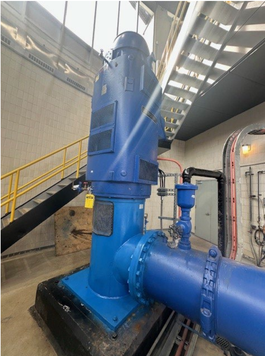
Figure 6: Low lift pump #1 after rebuild
